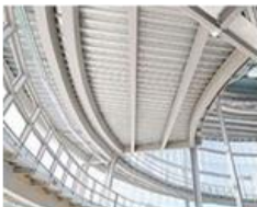
Structural Roof Deck
