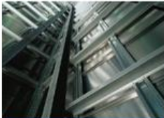
Purlins and Cladding Rails
