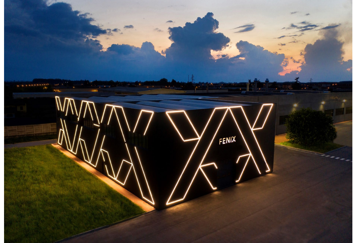
FENIX Factory view at night
