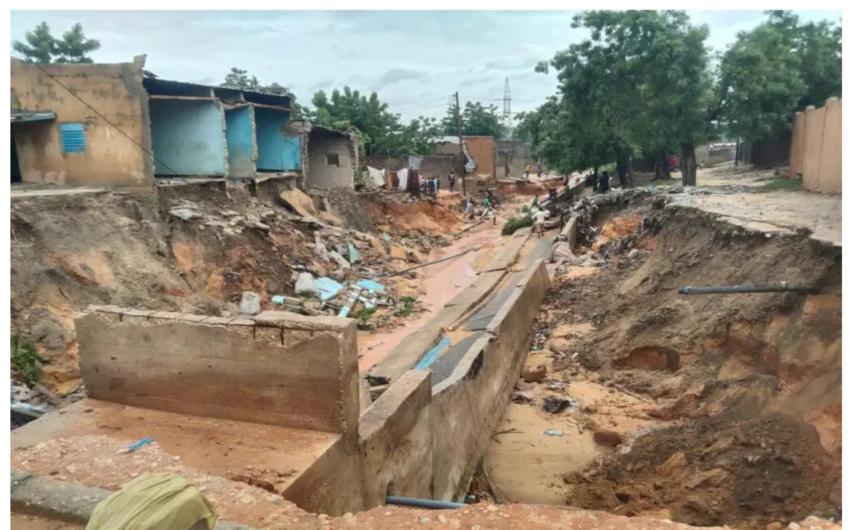
Photo 1. Houses destroyed by the flood of August 20, 2024 in the Maradi region
