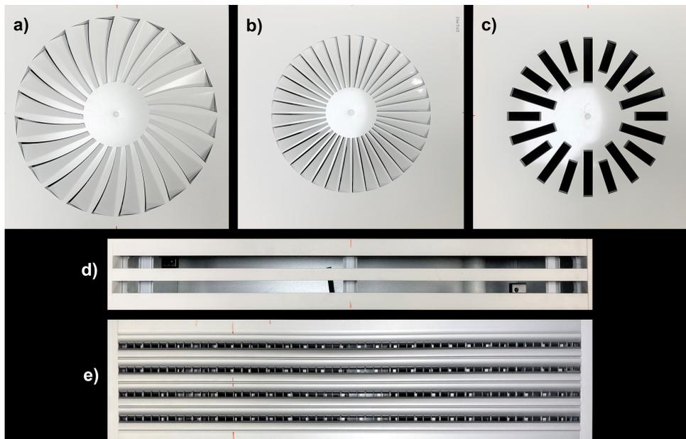
Figure 1: Selected air diffusers: a) swirl diffuser from TROX, b) swirl diffuser DTQ from Wildeboer, c) swirl diffuser DXQ from Wildeboer, d) slot diffuser from TROX, and e) slot diffuser from LTG.
