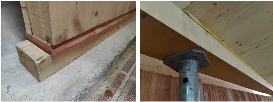
Figure 4: Wall support (left) ceiling support (right)
