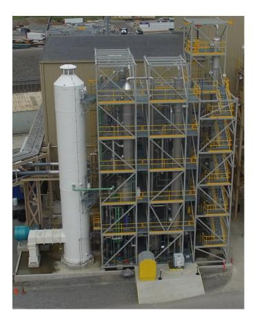
UKy-CAER 0.7 MWe small pilot scale  $CO_2$  capture facility located at Kentucky Utilities E.W. Brown Generating Station in Harrodsburg, Kentucky. (Funded under DE-FE0007395). Stats/specs: 0.7 MWe ~1300 acfm flue gas
