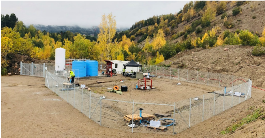
Figure 2: The new ECCSEL Svelvik CO 2 Field Lab not far from Oslo, Norway.
