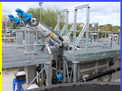
NIEA had issued an enforcement notice on the works therefore the primary driver for the scheme was to ensure the plant can treat the new FFT of 15.5 l/sec by replacing the MBRs with new back washable membranes with a higher membrane packing density and are much more efficient than the existing membrane modules in all respects.
