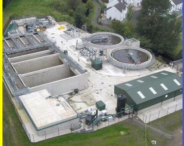
4 pumping stations, Emergency Storage Tank, Inlet Screening works, Aeration Lanes, Final Settlement Tanks, Sludge Processing Facility and associated Holding Tanks, Control Building and 2 nr Control Kiosks. A phased construction programme was required to maintain operation and treatment from the existing plant during construction of the new works
