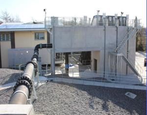
approximately 1,530. Works included demolition of the existing 6mm inlet works whilst using some of the existing structure to complete a new purpose built reinforced concrete Structure to hold 3 No 250 l/sec rated Screw Pumps working in Duty/Assist/Standby arrangement. With new flow balancing and control functions the downstream processes are better equipped to process the receiving flows and loads. New MCC & SCADA controls allows for full automatic operation and monitoring.
