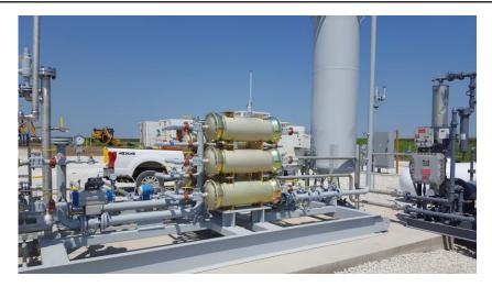
Raw biogas (64% CH<sub>4</sub>, 35% CO<sub>2</sub> is cleaned to >96% CH<sub>4</sub>
