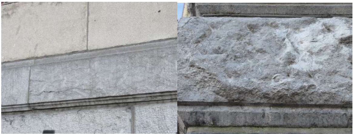
Plinth Rijksmuseum: Carboniferous limestone showing brachiopod shells (photo right). Above the blue limestone occurs cream colored ashlar of Upper Jurassic Euville limestone (photo left)
