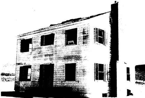
1.7 psi vs Wood frame house. Badly damaged but still standing. Flying debris likely fatal, but basement safe.
