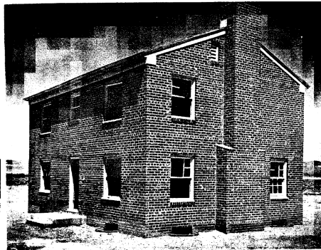
1.7 psi vs Brick house. Badly damaged but still standing. Flying debris likely fatal, but basement safe.
