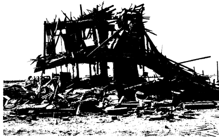
5 psi vs Brick house. House levelled and partially collapsed into basement.
