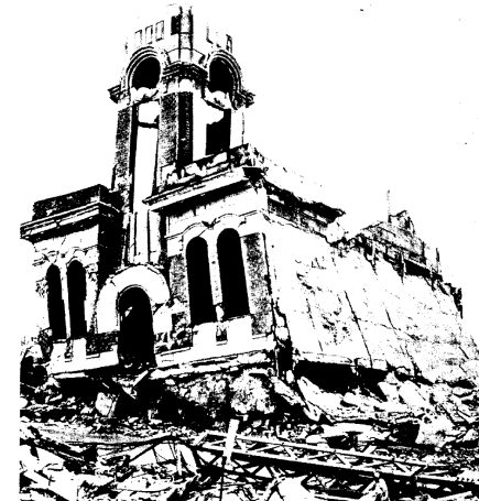
17 psi vs Steel + Reinforced concrete building. First story collapsed dropping second story to ground.
