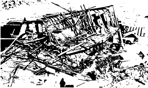
5 psi vs Wood frame house. House levelled but limited breakthrough to basement. Reasonable survival chance in basement.
