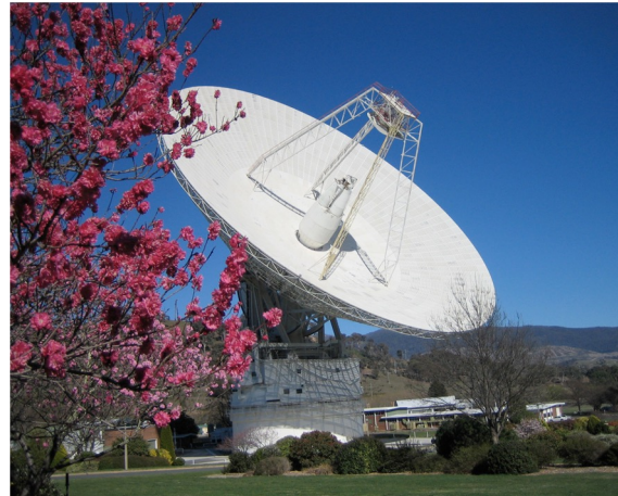
Southern Hemisphere Asteroid Radar Project Canberra DSS-43 (DSN) 70 m antenna, 80 kW transmitter, 4 cm wavelength (C band) + Australia Telescope Compact Array
