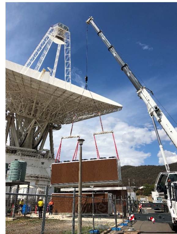
Hybrid Coolers Installation
