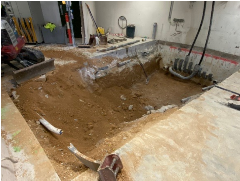
Trench Excavation for Substation
