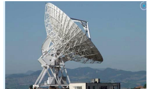
European Demonstrations Madrid DSS-63 (DSN) 70 m antenna, 20 kW transmitter, 4 cm wavelength (C band) + Medicina Antenna
