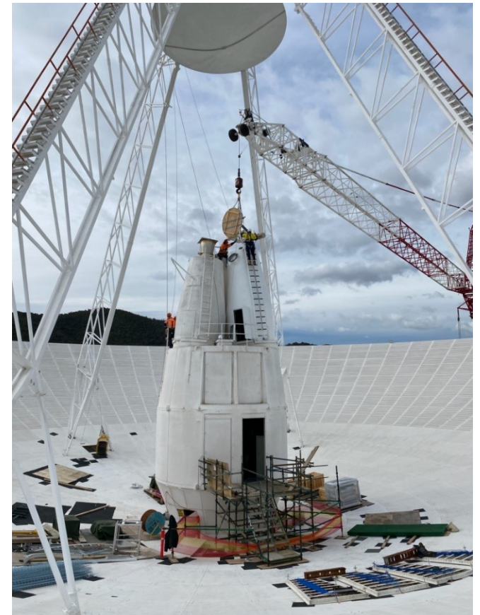
Canberra TT&C Cone Replacement
