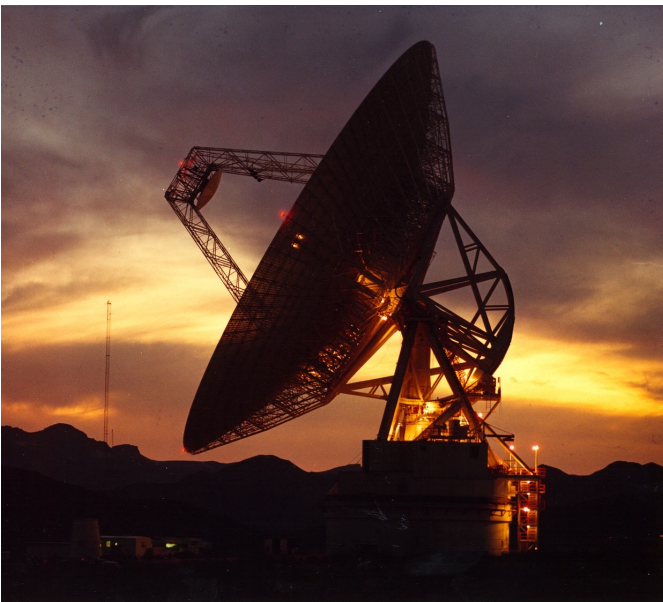
Goldstone Solar System Radar (GSSR) 70 m antenna, 450 kW transmitter, 3.5 cm wavelength (X band)
