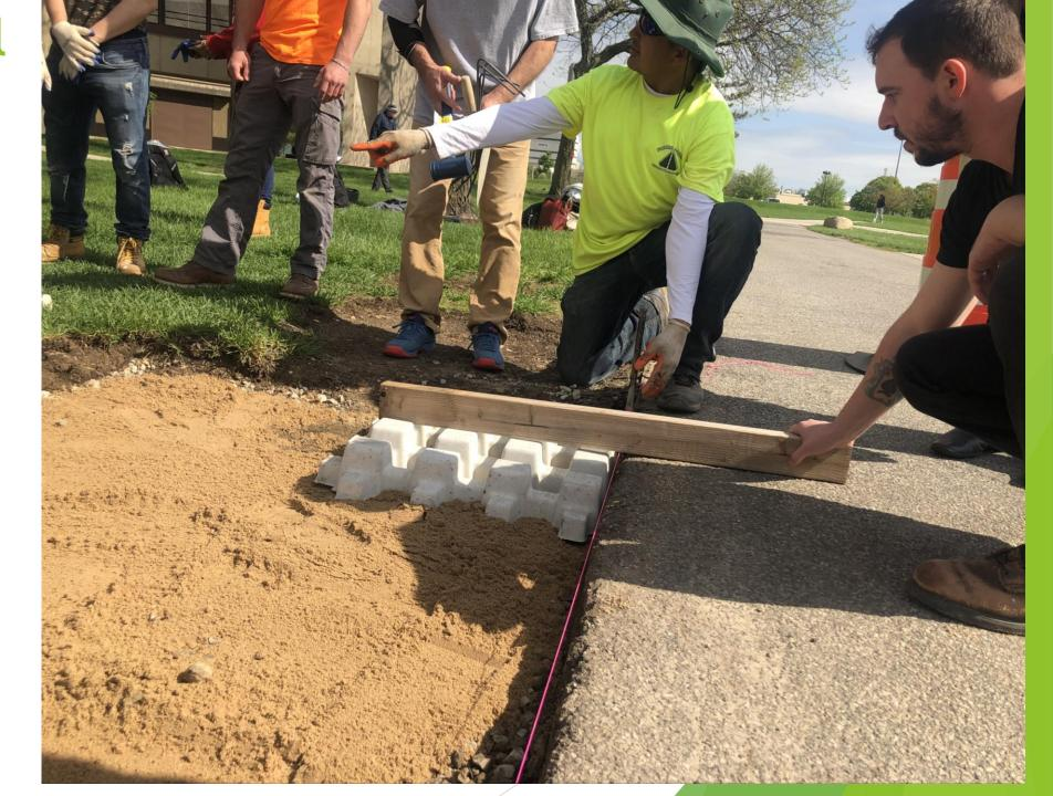
Placing more sand and smoothing out to make sure first paver is level.
