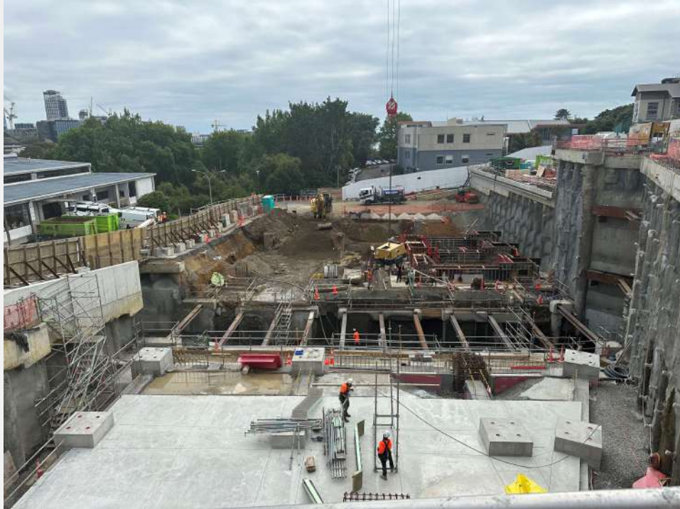
ZONE A SLAB ON GRADE POURED
