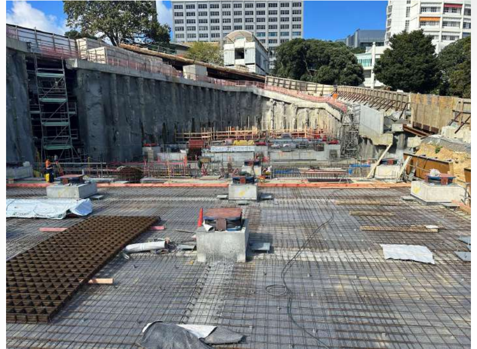
ZONE B SLAB ON GRADE PROGRESSING
