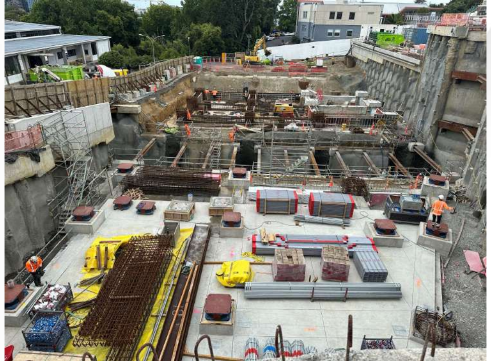
ZONE B GROUND BEAMS AND FORMWORK BEING INSTALLED
