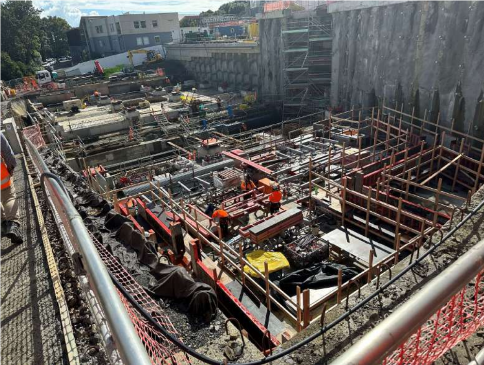
ZONE B SLAB ON GRADE POURED
