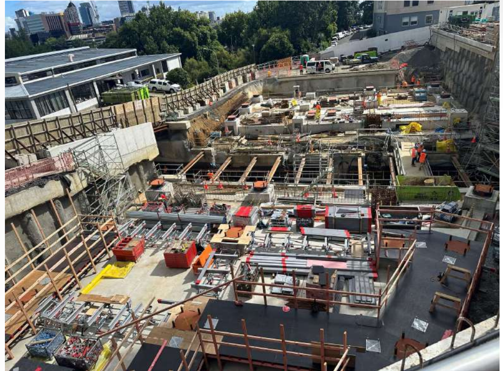
ZONE B ISOLATORS INSTALLED, TUNNEL REO/ STRUTS PROGRESSING
