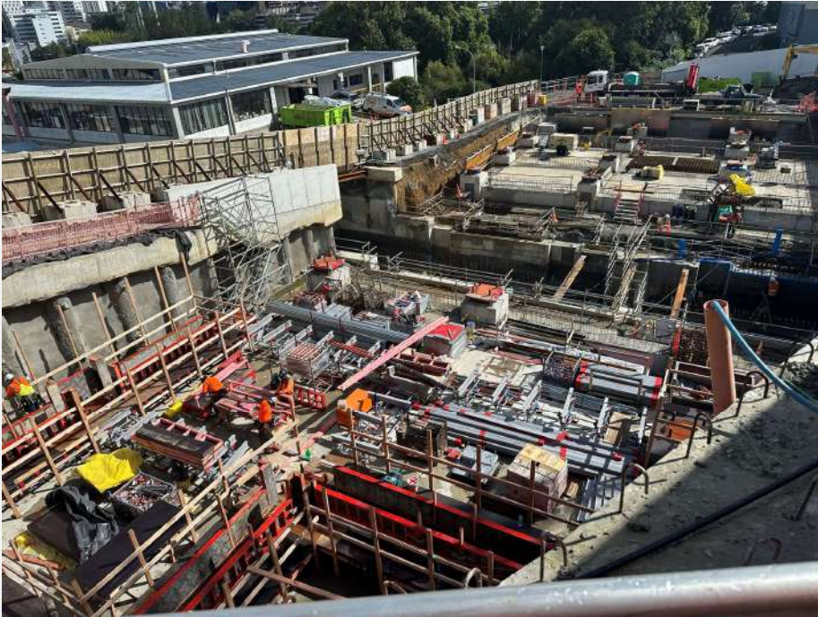
ZONE A ISOLATORS INSTALLED, TUNNEL REO PROGRESSING
