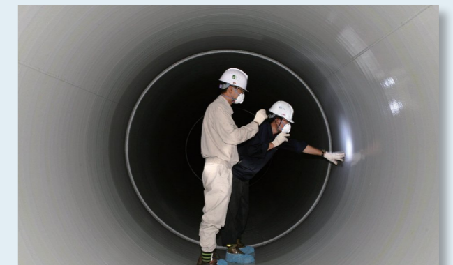
Examining of lining condition
