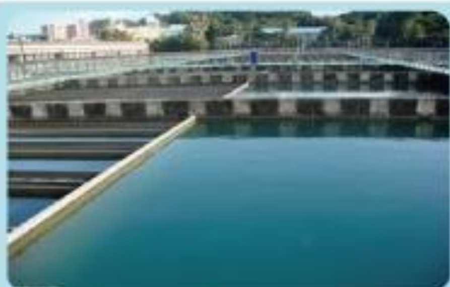
Water Treatment- pH, Free Chlorine, Turbidity
