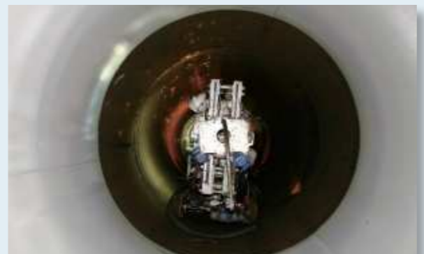
Lining of the insides of the pipes
