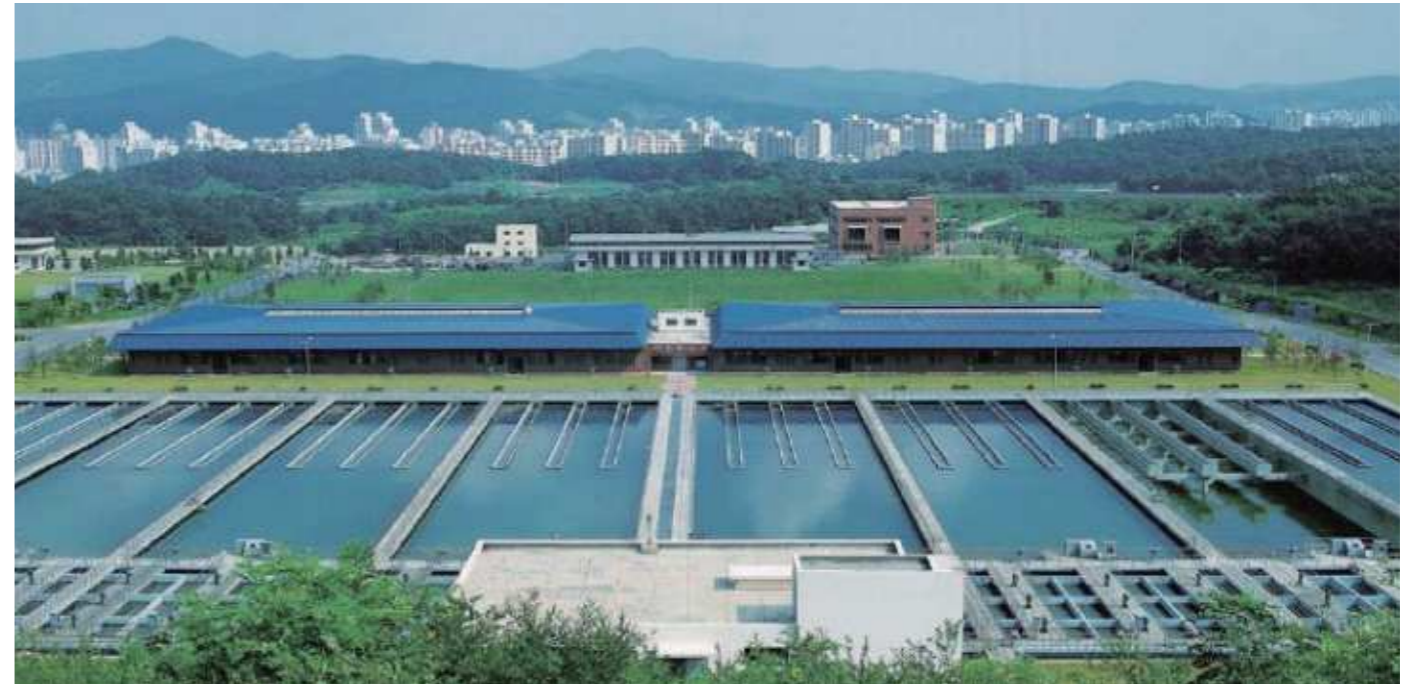
Seongnam Water Treatment Plant
