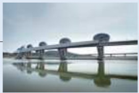
Operation & maintenance of hydraulic structures in rivers
