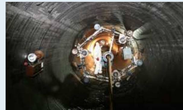
Removal of the residual painting materials
