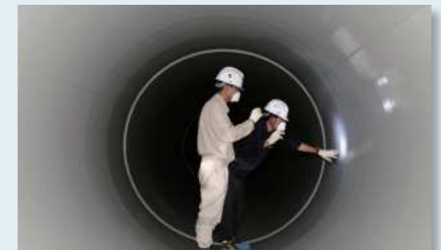
Examining of lining condition
