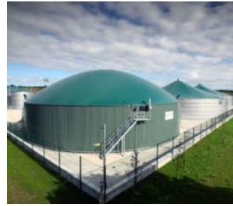
Biogas energy plant
