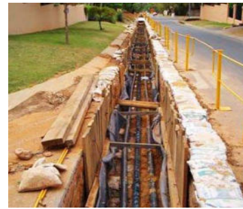
Integrated utility relocation
