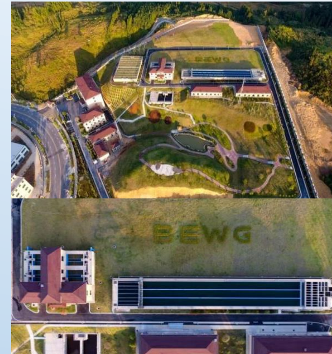
Rucheng Second Tap Water Plant built under this PPP project
