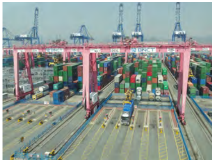
Automated Stacking Crane(ASC)
