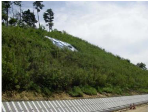
Slope protection by greening mats
