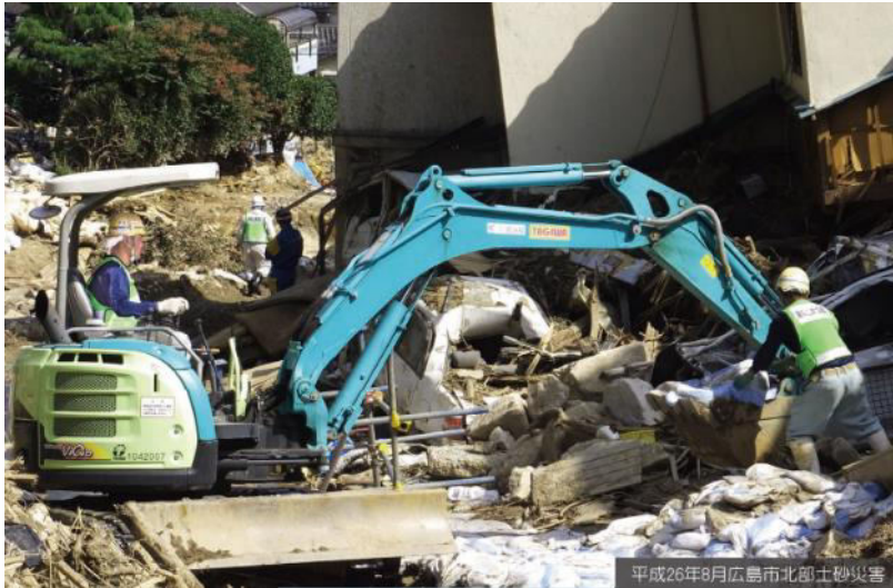
Local construction companies working for debris removal
