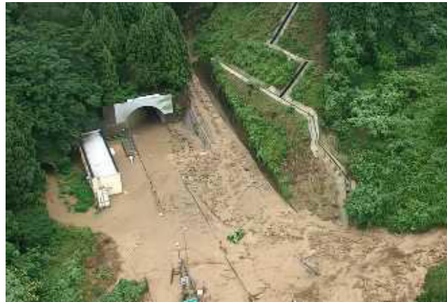
Mudslides by torrential rain in August, 2022
