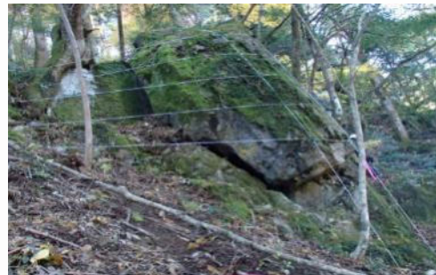
Rock stabilization by wire rope
