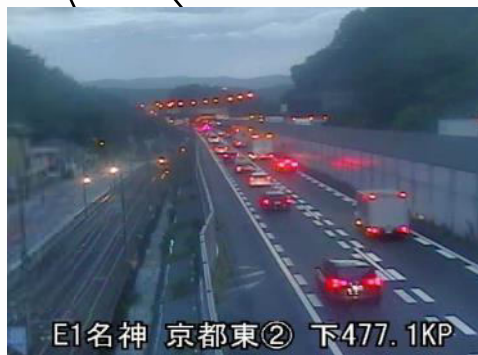
Passable E1 Meishin Expressway (No damage)
