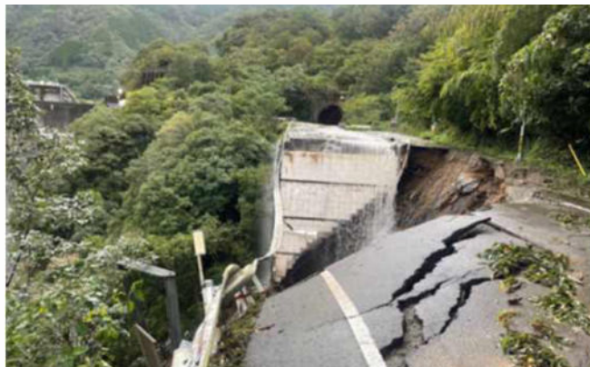
Road collapse after Typhoon Nanmadol in September, 2022
