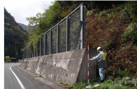
Rockfall protection wall/fence
