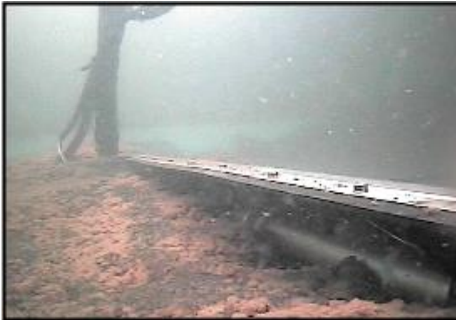
● Before removing sludge
