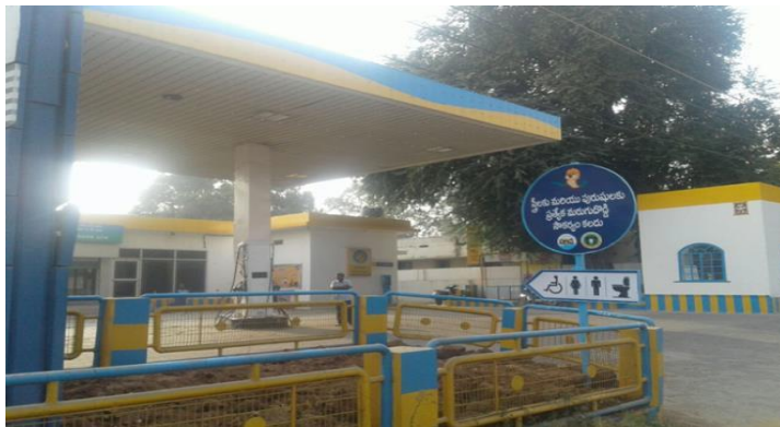
Toilets at Fuel Stations
