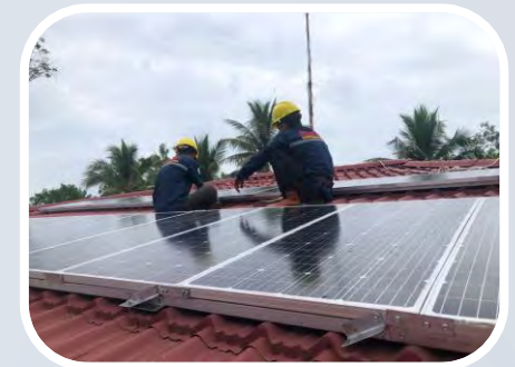
Solar Power Plant Installation
