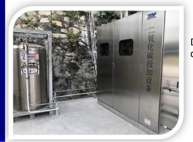
The carbon dioxide dosing system is made up of Dewar storage system, pressure tank system, pH detection system and automatic control system.
