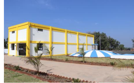
Clean water storage
