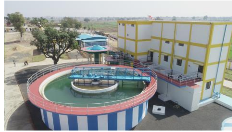
Treatment and SCADA
