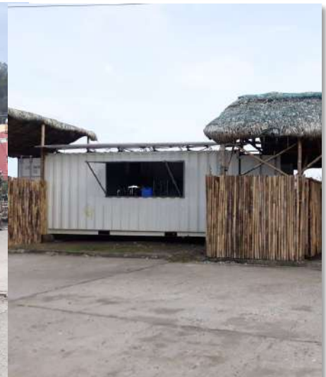
NXTLVL Hydra Site
