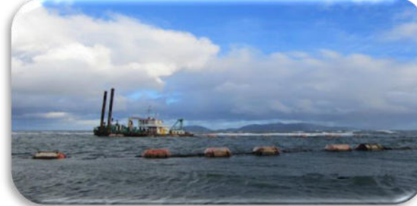
Dredging ( Administered by FPCL – Work carried out by private contractor )
