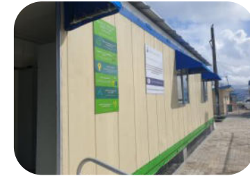
Carbon neutral facility at Muaiwalu 2
