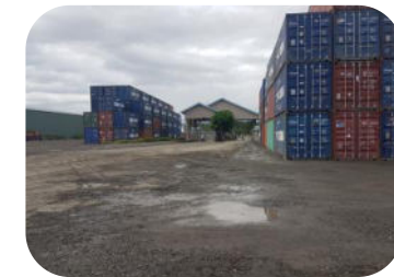
Lautoka Yard 4 project
