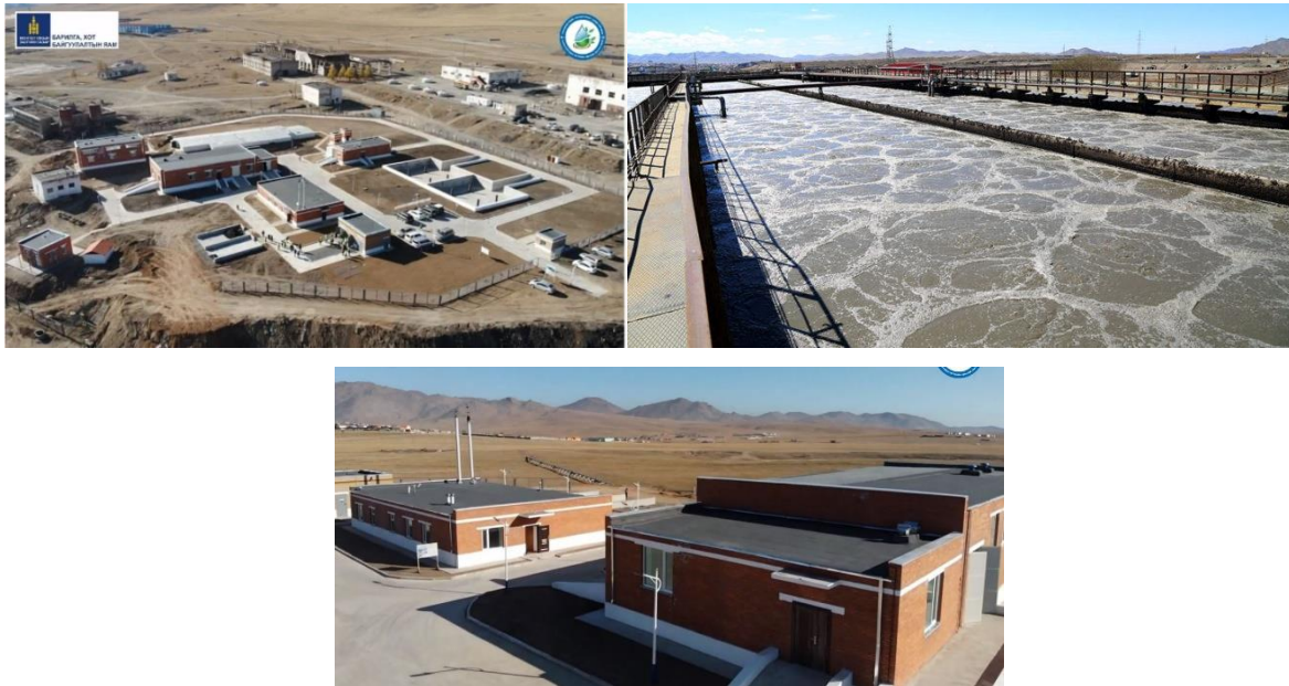
Figure 14. Photos from new water supply and sanitation infrastructure for residents of Dalanzadgad Soum
