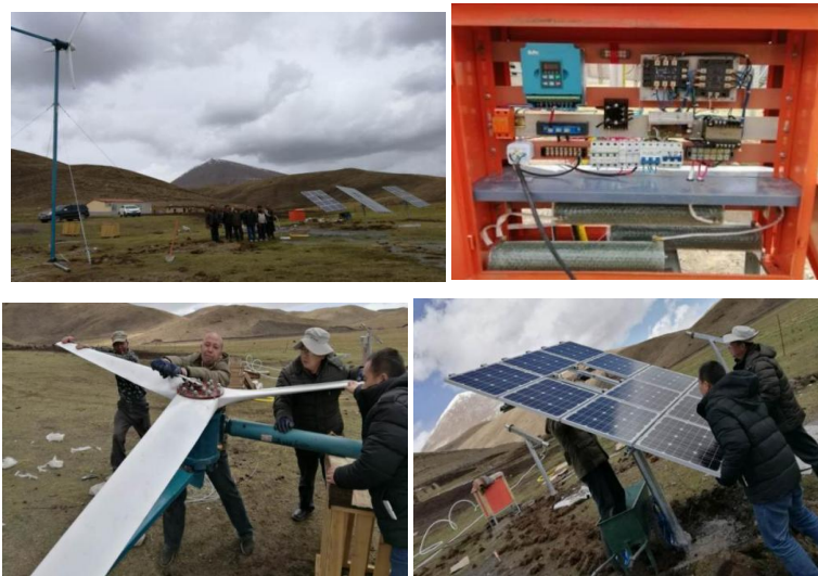
Figure 11. Photos of the demo project in Gangchagongma Village
