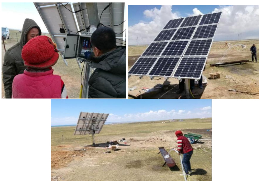
Figure 9. Photos of the demo project in Jiaoshikexiuma Village
