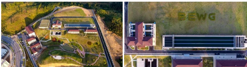
Figure 12. Rucheng Second Tap Water Plant built under this PPP project
