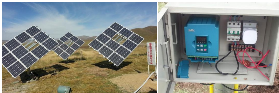
Figure 7. Photos of the demo project in Huanlunxiuma Village
