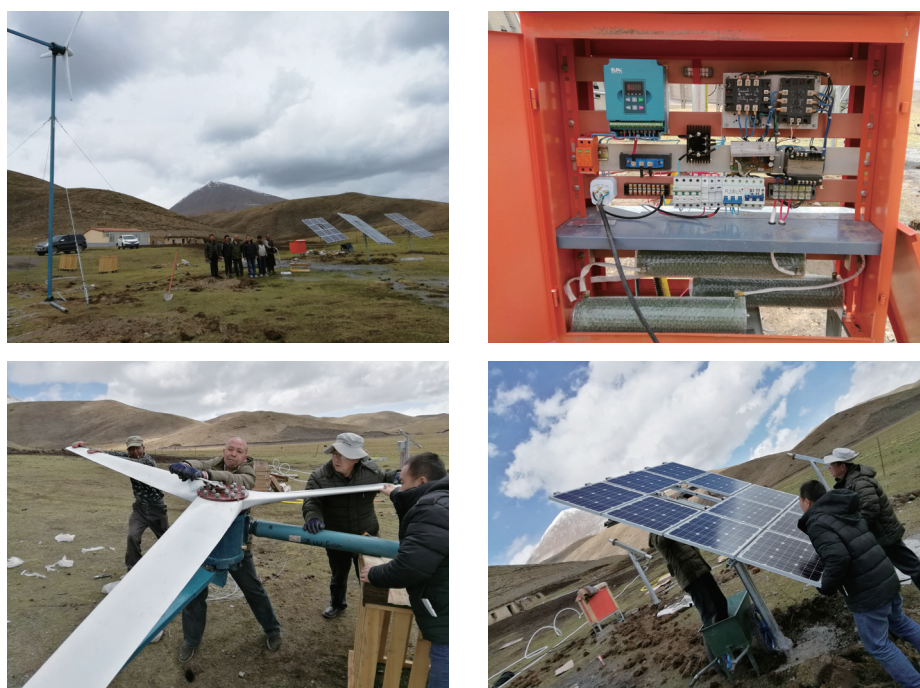
Figure 11. The Demonstration project in Gangchagongma Village
