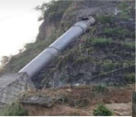
Turbine water is fed through pipe from distance location and height.
