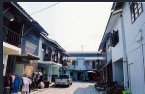
CODI Upgrading project
