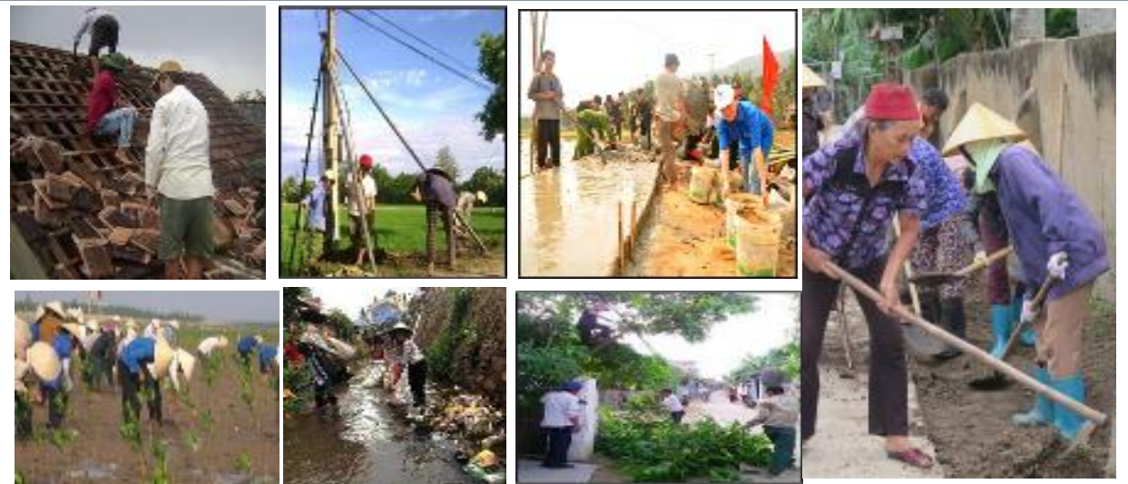
2) Raise community awareness on CC & Improve community-led climate-resilient infrastructure
