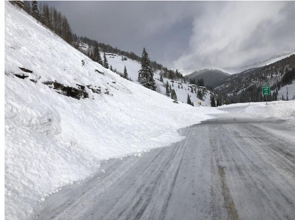
Figure 1. An example of small avalanches running into the inside lane. In areas with lower traffic volumes and slower speeds, drivers can navigate avalanches like these by taking turns driving in the open lane. Events like this can, however, slow or stop traffic under other large avalanche paths which may be an intolerable situation in some areas.
