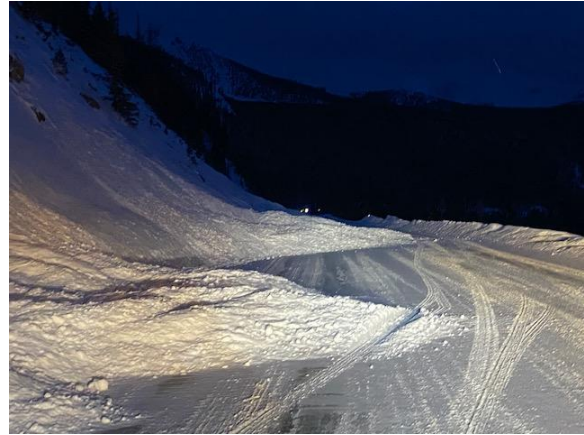
Figure 3. Small avalanches in areas where the avalanche path plunges to the road can easily put debris in the outside lane constituting an intolerable event.
