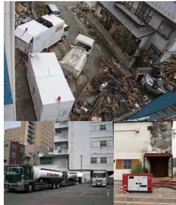
Power supply vehicles, fuel tankers, and emergency generators provide temporary power to telecom facilities.
