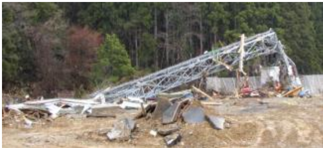
Cell site destroyed by tsunami in Rikuzen-takata
