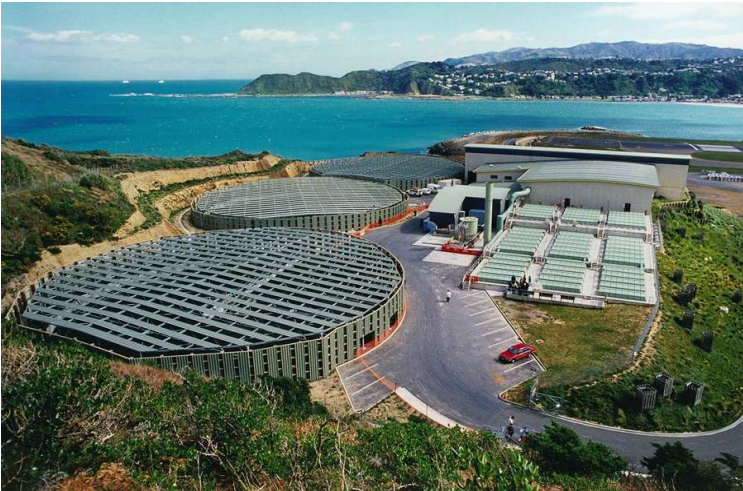
Moa Point Sludge Minimisation Facility
