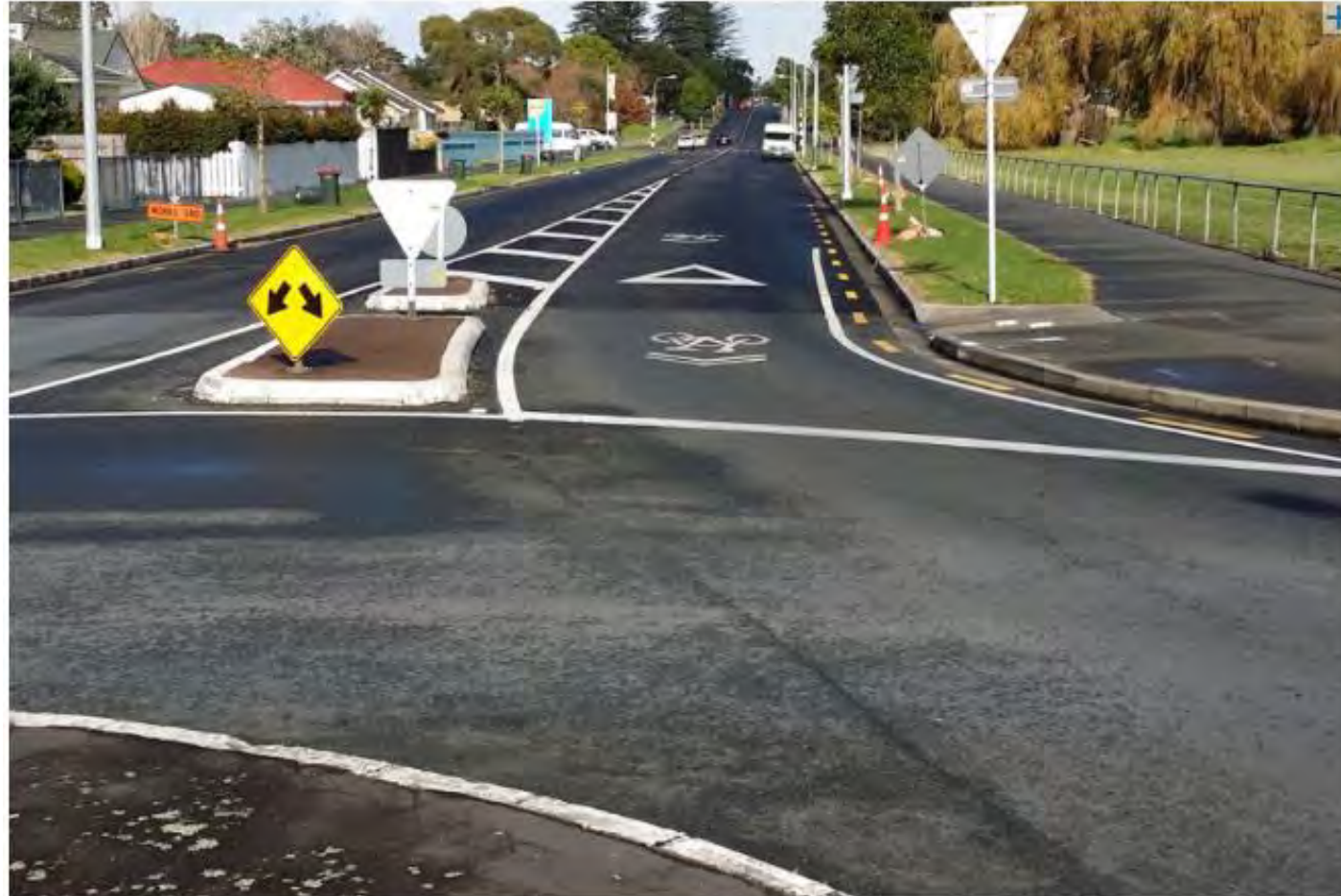
Sharrow markings to indicate that cyclists share the lane, Elstree Ave/Taniwha St, Auckland (Glen Koorey)
