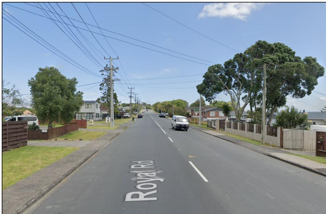
Figure 5: Typical Urban Corridor Recommended for Upgrade
