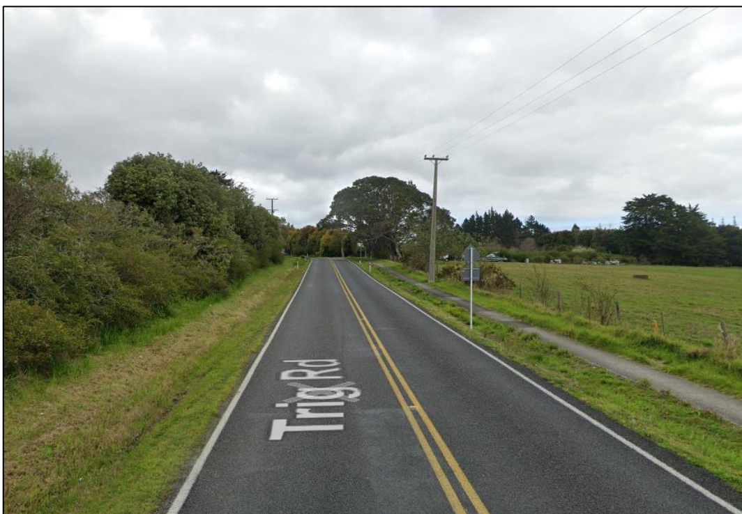
Figure 6: Typical Rural Corridor Recommended for Upgrade
