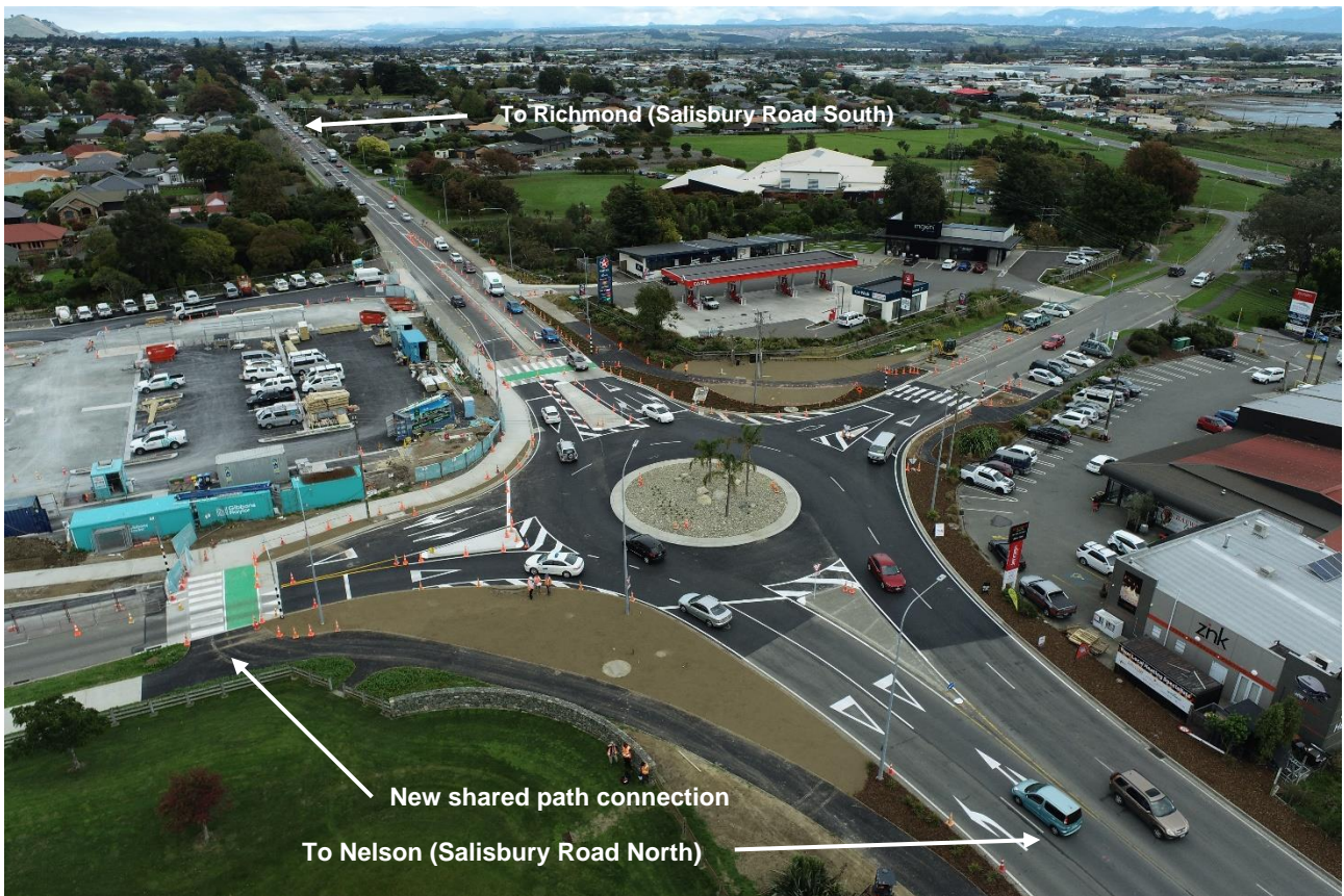
Figure 5: Aerial photo of the completed upgrade
