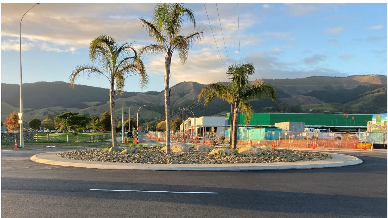
Figure 6: View of the roundabout from the ground
