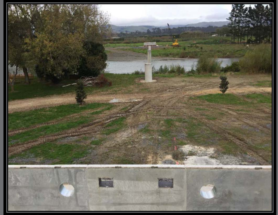
Abutments and piers completed – looking from city side
