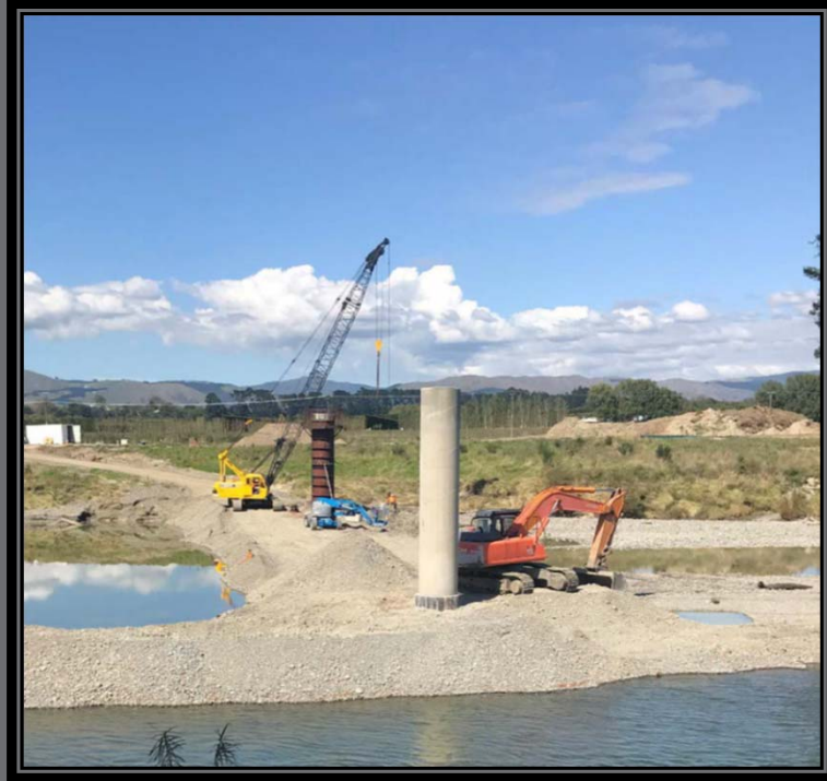
Pier construction from causeway in river
