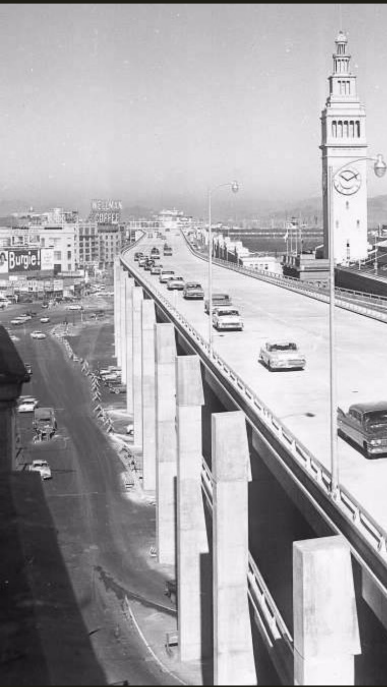
San Francisco, Embarcadero Freeway
