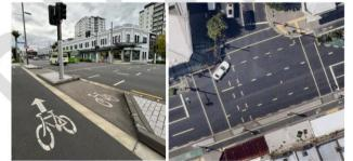
Figure 25: Separator gap waiting space for cyclist turning right on T-Intersection of Karangahape Rd and
