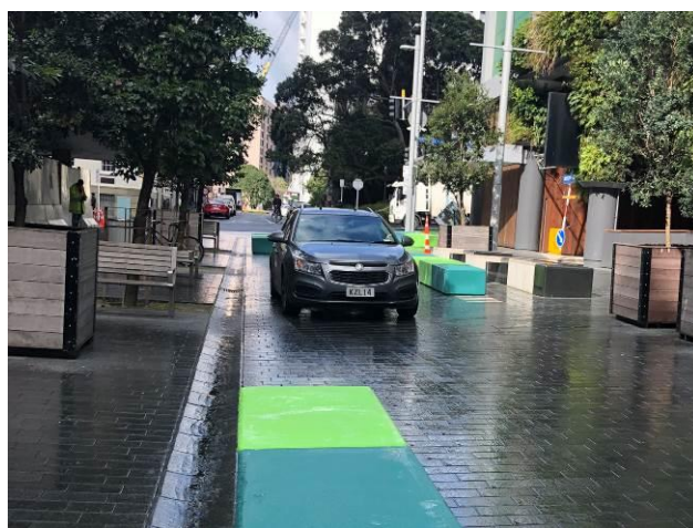
Figure 11: Federal Street chicane and tree planters
