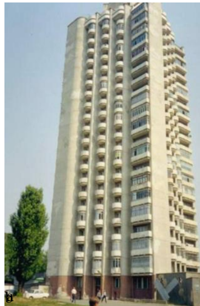
Figure 2. 24-storey building, alkali-activated BFS concrete, Lipetsk, Russia, 1986~1994 (P. V. Krivenko, 1994)
