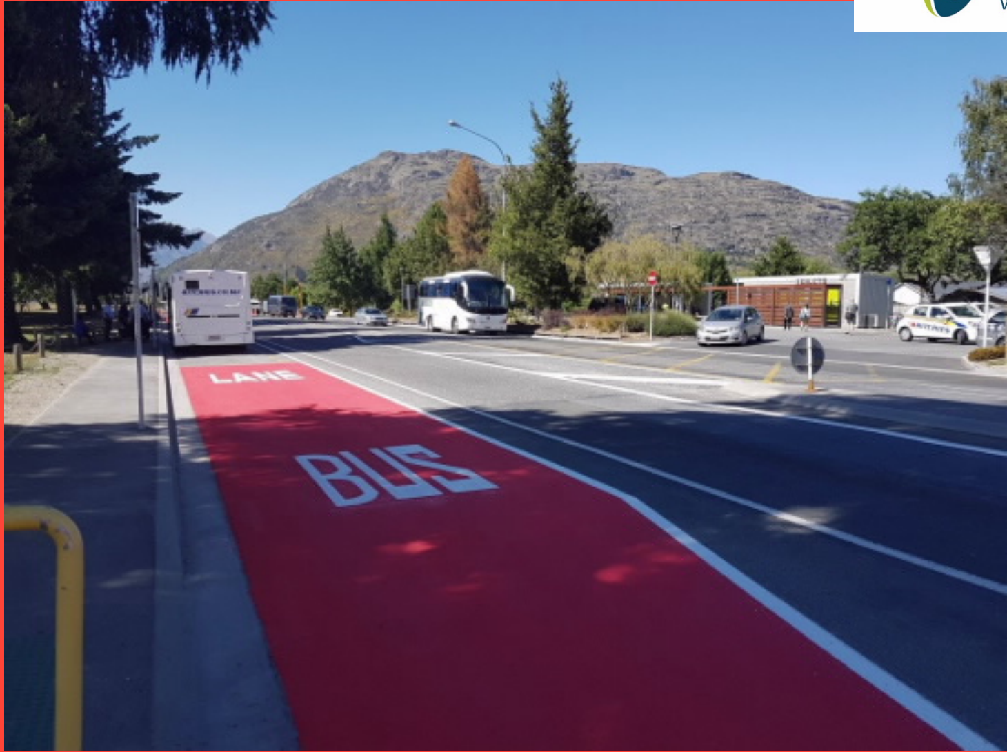
Planning the SH6 Corridor in Queenstown
