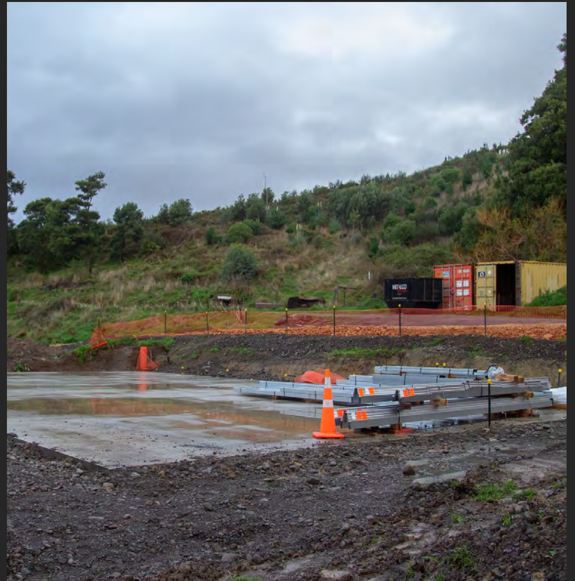
June 2021- Concrete slab is down
