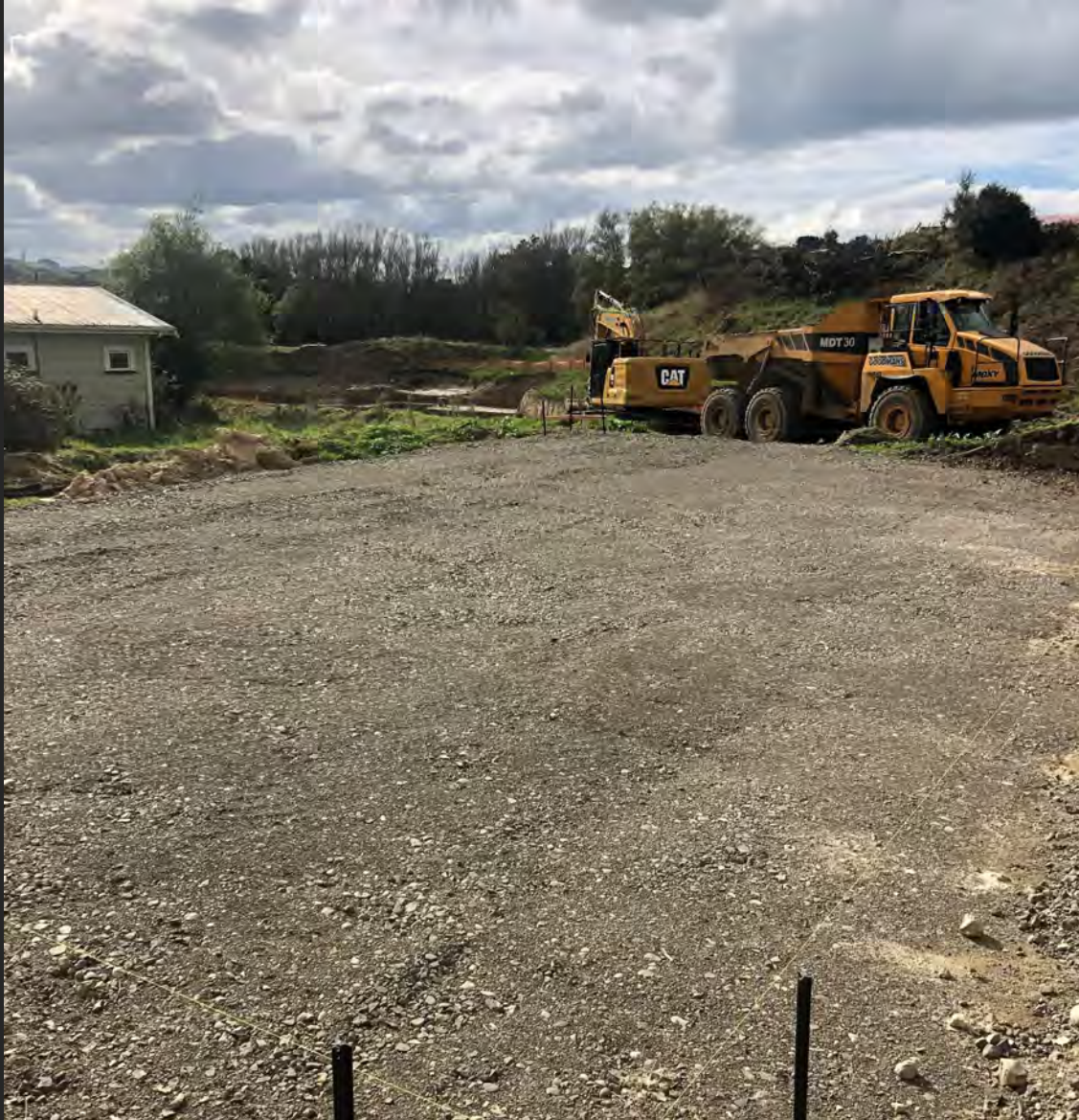
May2021- Lab earthworks starts
