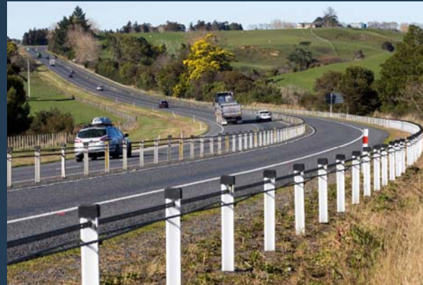
Flexible barriers, Waikato Expressway
