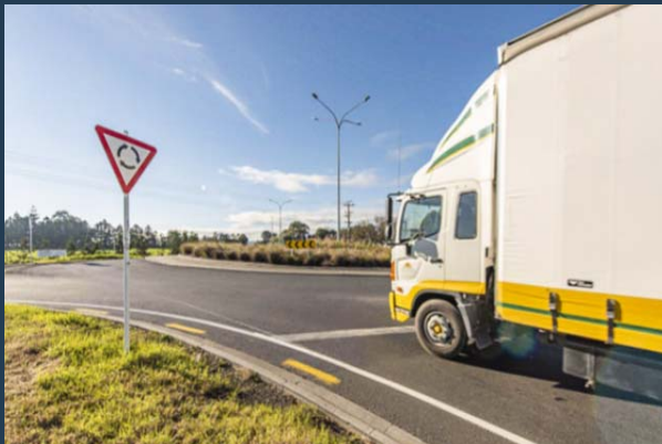
Rural roundabout, Glenbrook and Kingseat
