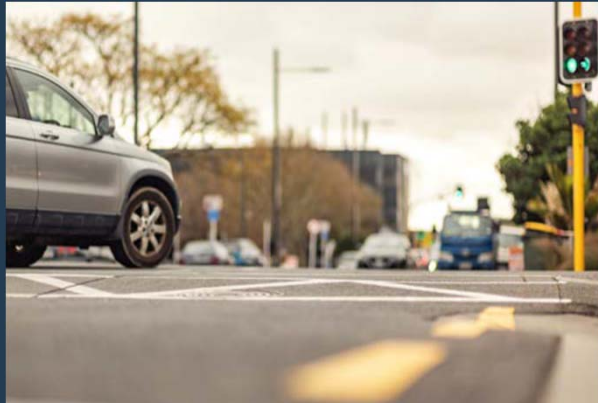
Raised table intersection on Great North Road
