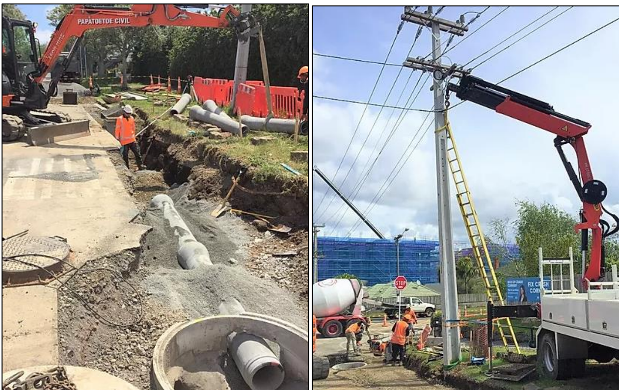
FIGURE 5: STORM WATER WORKS
