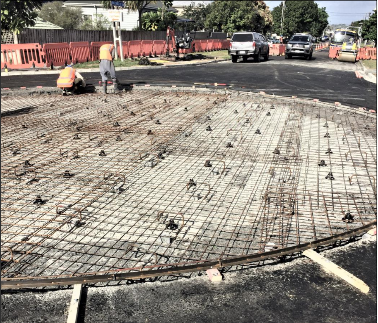
FIGURE 4: FULL TRAFFIC CLOSURE - ROUNDABOUT ISLAND CONSTRUCTION
