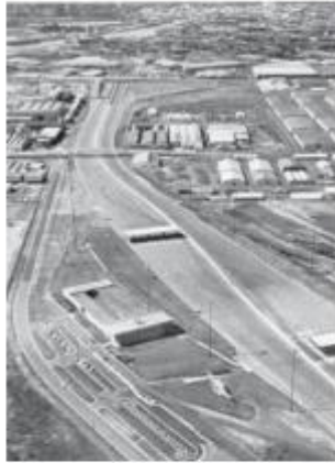
West Gate Freeway expansion
