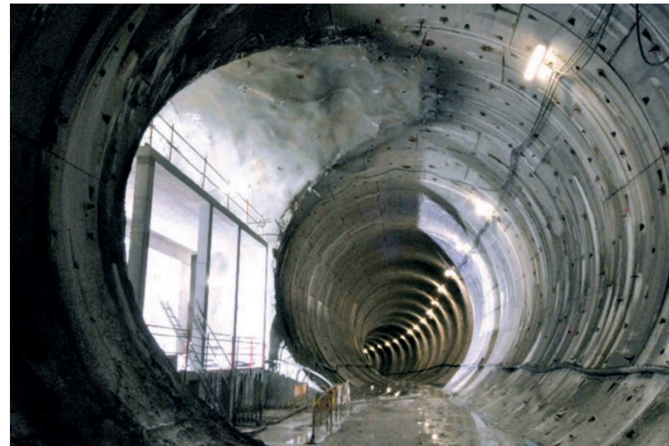
Barcelona Metro Line 9
